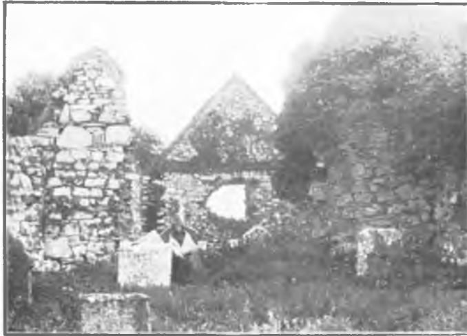
INTERIOR OF RUINS OF TULLYLEASE CHURCH SHOWING CHANCEL.
