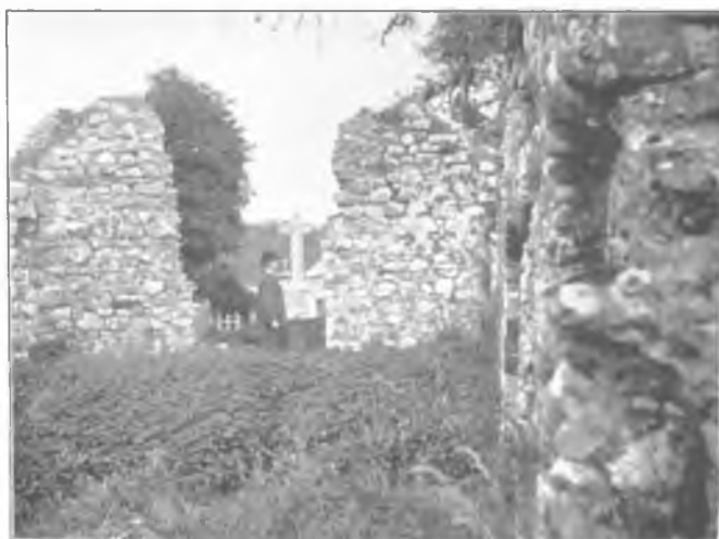
INSIDE THE RUINS OF KILDORRERY CHURCH.
