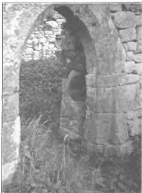
FONT IN DOORWAY OF RUINS OF KILDORRERY CHURCH.
