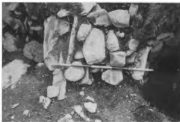
2. Roof of Passage.
