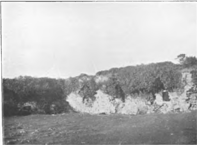
NORTH WALL OF BAWN—INTERIOR. BALLINACOLLIG CASTLE.
