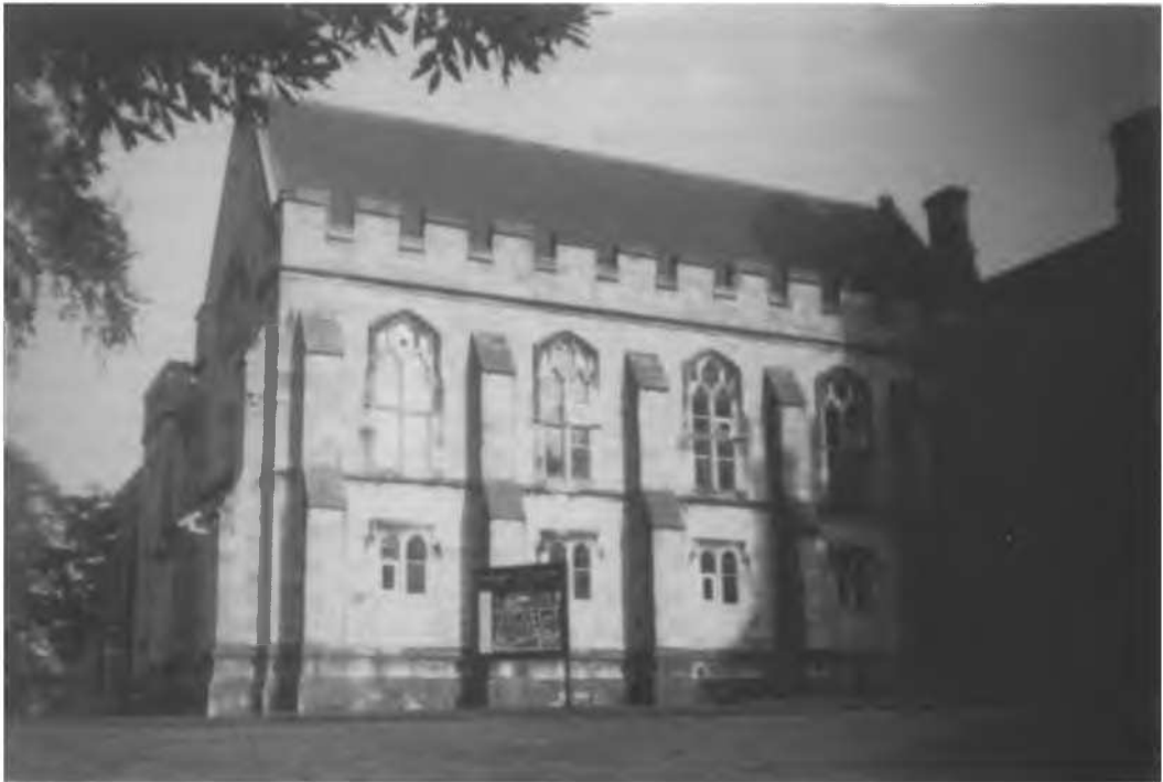
AULA MAXIMA, ADJOINING OLD LIBRARY BUILDING, QCC
