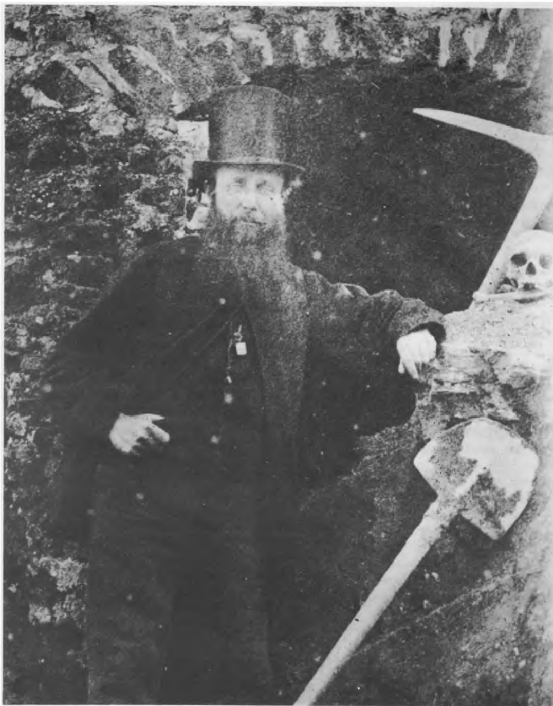
CAULFIELD EXCAVATING A VAULT AT ST FIN BARRE'S, CORK
